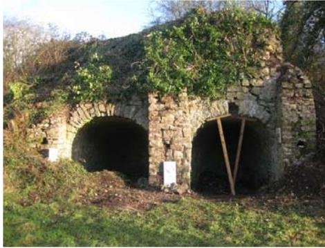
into the stone work and it is clear to see that these roots are slowly prising apart the stones. While we are waiting for the poison to do its work we have set up timber supports to brace the right hand arch to make it safe and hopefully to prevent any further collapse of the fragile masonry. We have also cleared the large Crack Willows from the adjacent pond, opening up the view of the former limestone quarry face at the rear.
