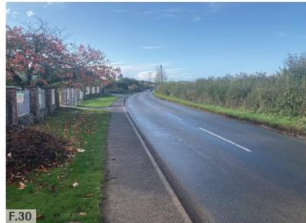
Figure 30: View south along Dormington Road.
