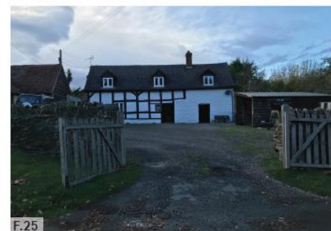
Figure 25: Detached property with associated outbuilding, featuring white render and timber beams. Properties are well spaced on generous plots.
