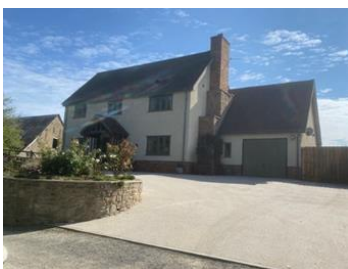
Garlands Lodge – new build
