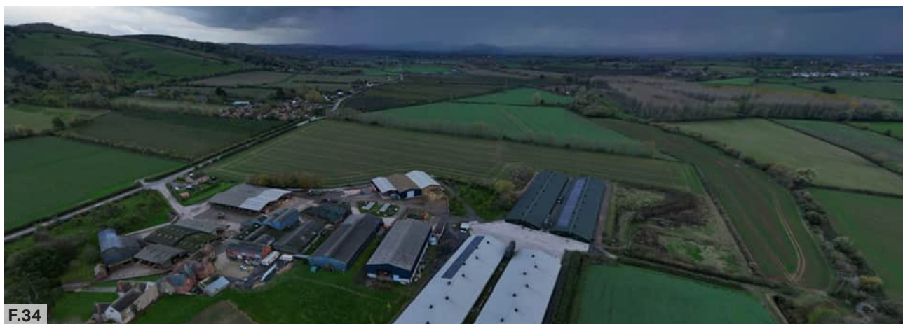
Figure 34: Aerial view of Claston Farm looking east along the A438. Source: DJ Audit https://www.google.com/maps/@52.0630336,-2.6069283,3a,75y,218.38h,69.32t/data=!3m8!1e1!3m6!1sAF1QipM77cCXPsVEC70NfW6SqH_xoCUyrCE7hVBHRqTu!2e10!3e11!6shttps:%2F%2Fh5.googleusercontent.com%2Fp%2FAF1QipM77cCXPsVEC70NfW6SqH_xoCUyrCE7hVBHRqTu%3Dw203-h100-k-no-pi0-ya86.13762-ro0-fo100!7i8192!8i4096
