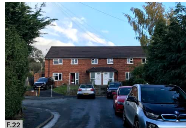
Figure 22: Terraced properties within the Sufton Rise estate.
