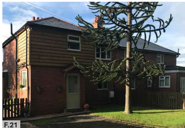
Figure 21: Semi-detached properties along Sufton Lane.
